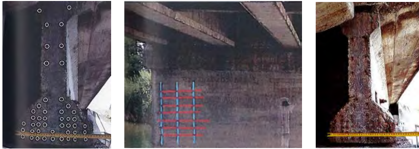
2018: DESTRUCTIVE AND NON DESTRUCTIVE TESTS
