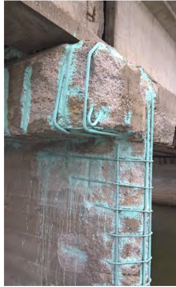
2019: PASSIVATION OF PIERS REINFORCING BARS
