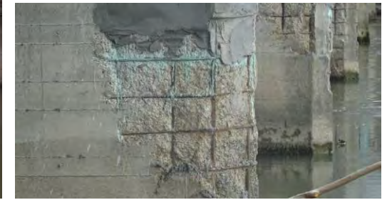
2019: PASSIVATION OF PIERS REINFORCING BARS
